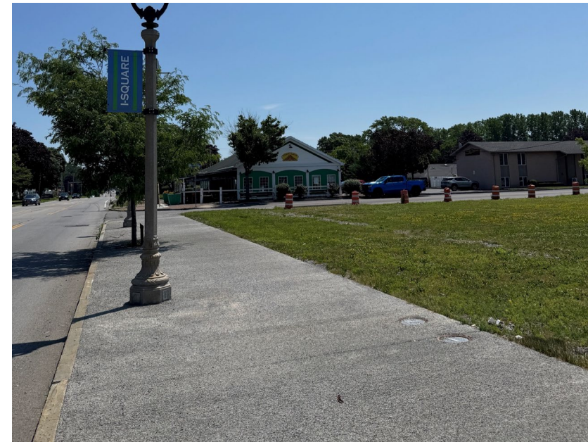
Concrete sidewalk, no buffer strip
