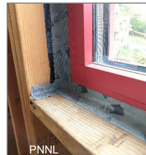
Weatherization + air sealing, vapor barriers
