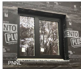
Window replacement, shading, films
